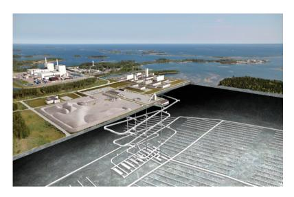
**Figure 9.3** The planned repository for spent nuclear fuel at Forsmark (image by Lasse Modin, courtesy SKB).
