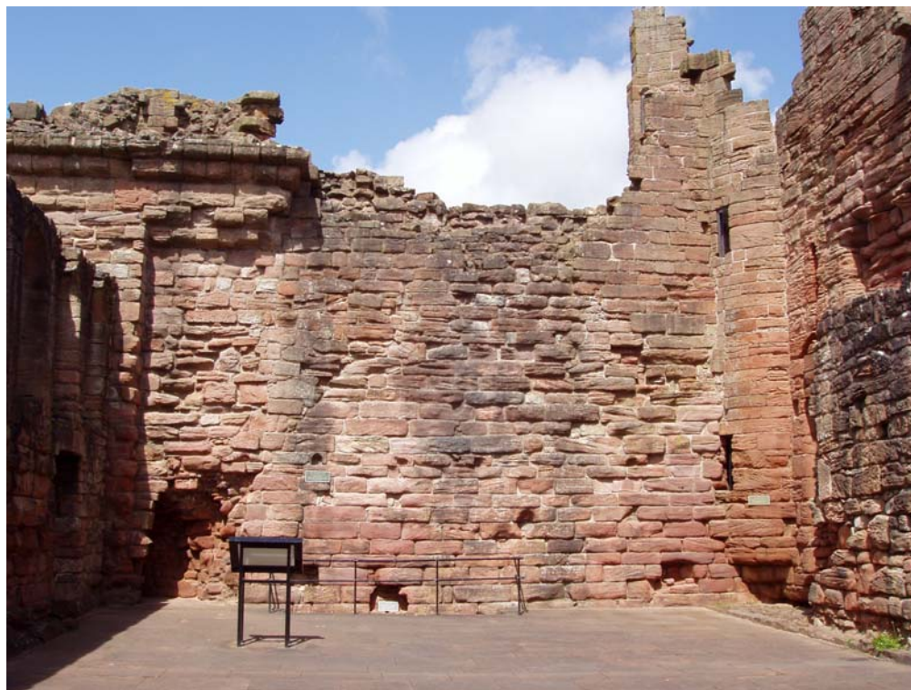
Bothwell Castle: Great Hall, north facing, interior view
