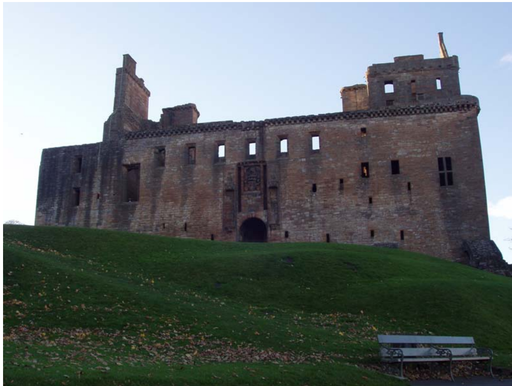
Linlithgow Palace, East Range, exterior view
