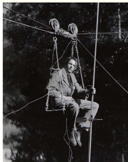
William McClean conducting a river flow test, River Garry, 1913.
