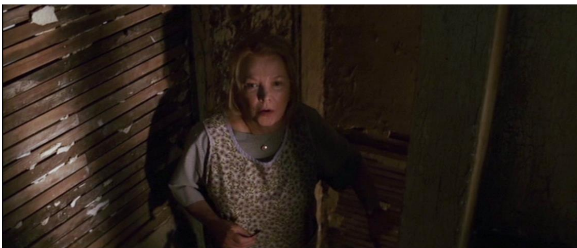
Figure 47: The dilapidated attic staircase.
