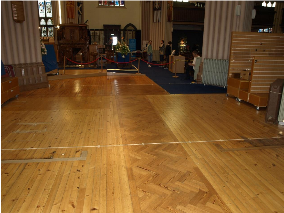
Figure 45: Survey Area 3, viewed from the North door. Tape 2 is in the foreground, tape 1 towards the South.
