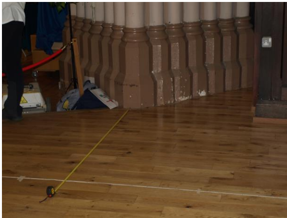
Figure B5: Pillar Measurement to end of tape not shown.
