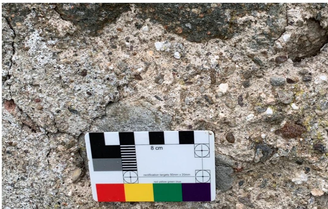
Figure 2.5. Lime inclusions, commonly in mortars mixed 'hot'.
