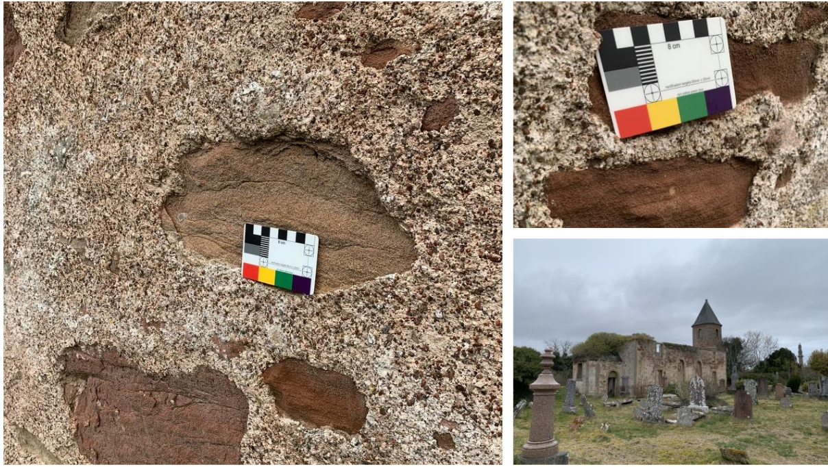
Figure 3.13. The Gaelic Chapel, c. 1783, Cromarty. FDC mortar surviving at the expense of the soft underlying sandstone.
