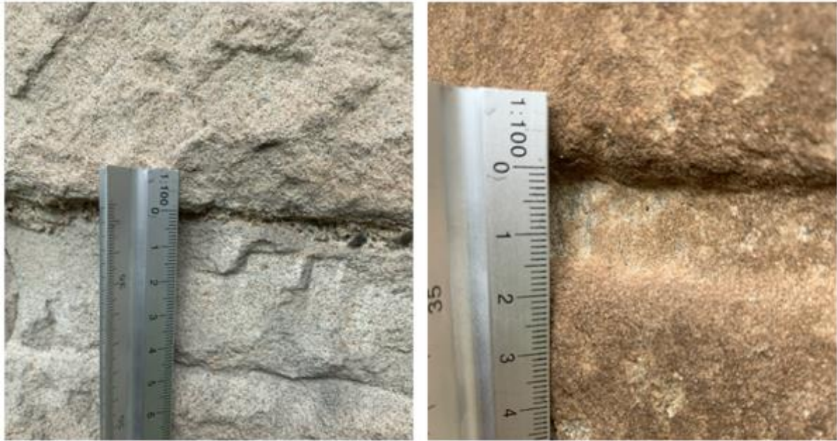
Figure 2.60. Left: the width of Playfair. Right: the chase width of Adam.
