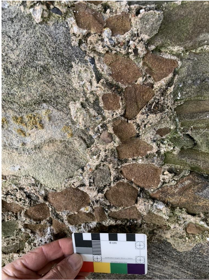
Figure 2.34. Fairburn Tower, Inverness Shire. Seventeenth-century packing out of wall surface. Closely packed wall face.
