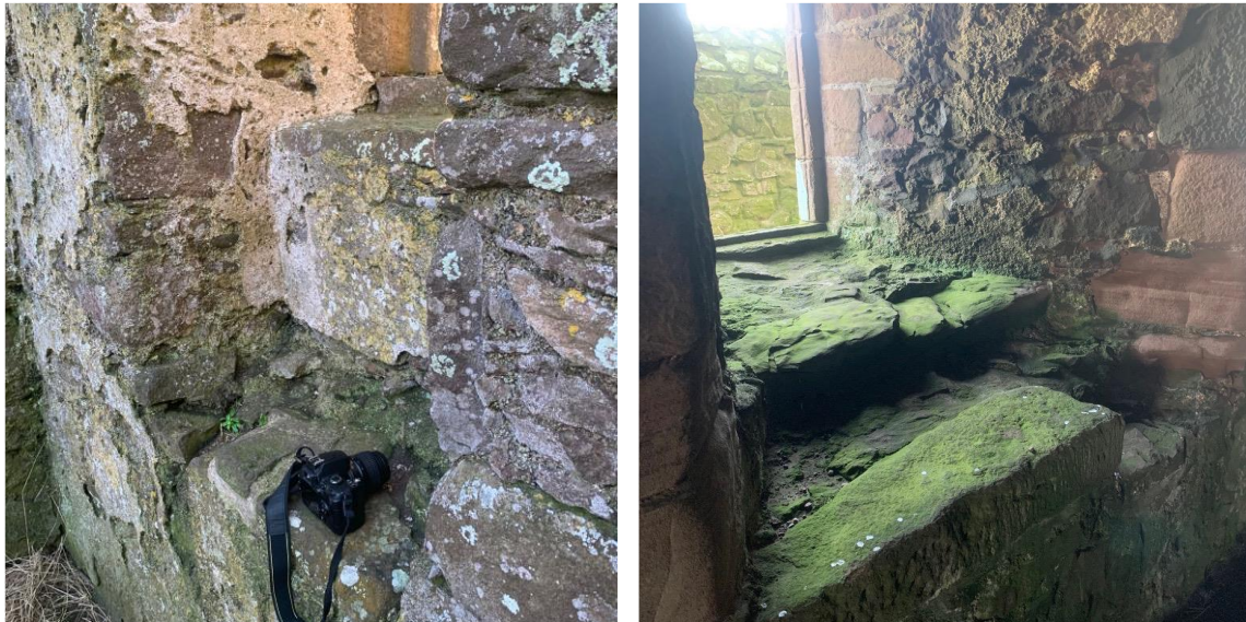
Figure 4.5. Dunnotter Castle. Seating area in the window opening allowing light in to undertake tasks rather than the view out.
