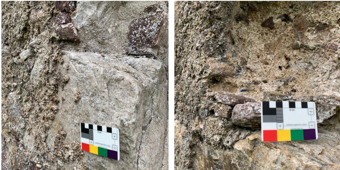
Figure 2.23. Left: Ardvreck Castle. Right: Calda House, Sutherland. Harl contiguous with the bedding mortar.
