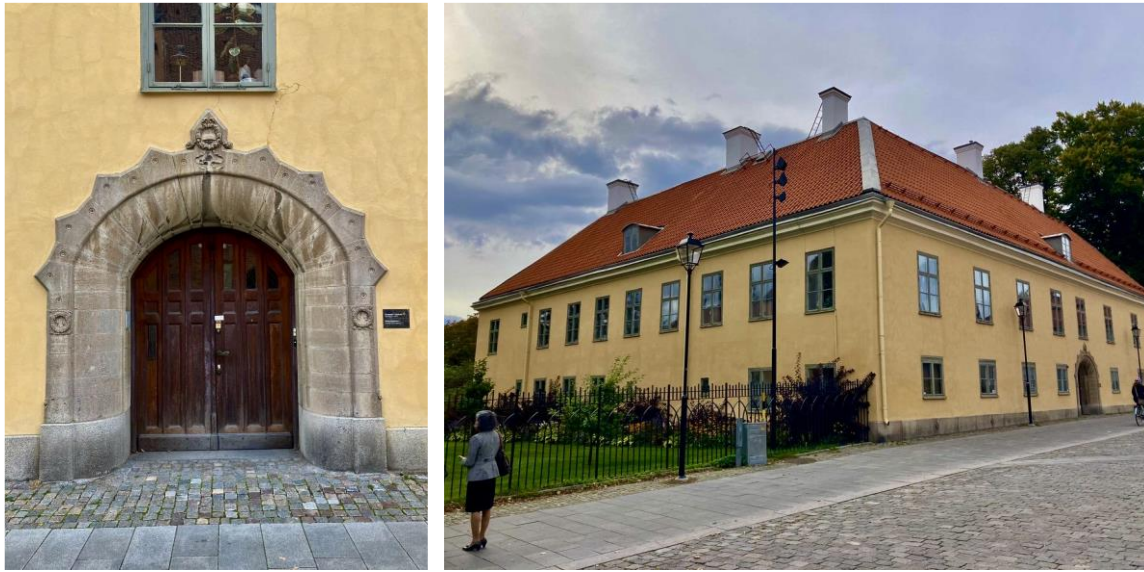
Figure 6.6 Västerås, Sweden. Plastered and limewashed buildings located next to the cathedral. Image credit J.P. Viktor.
