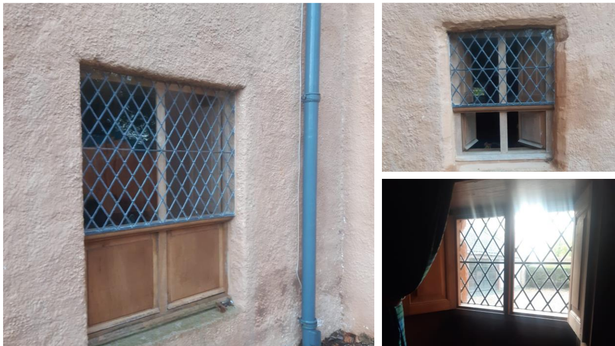
Figure 4.6. The shutterboard window providing light at the top and ventilation at the bottom.
