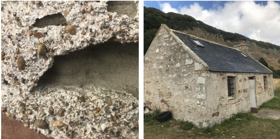
Figure 3.15. Geanies House salmon bothy, c. 1870, Fearn, Ross shire. Extreme weathering of sandstone while the weathered harl survives.
