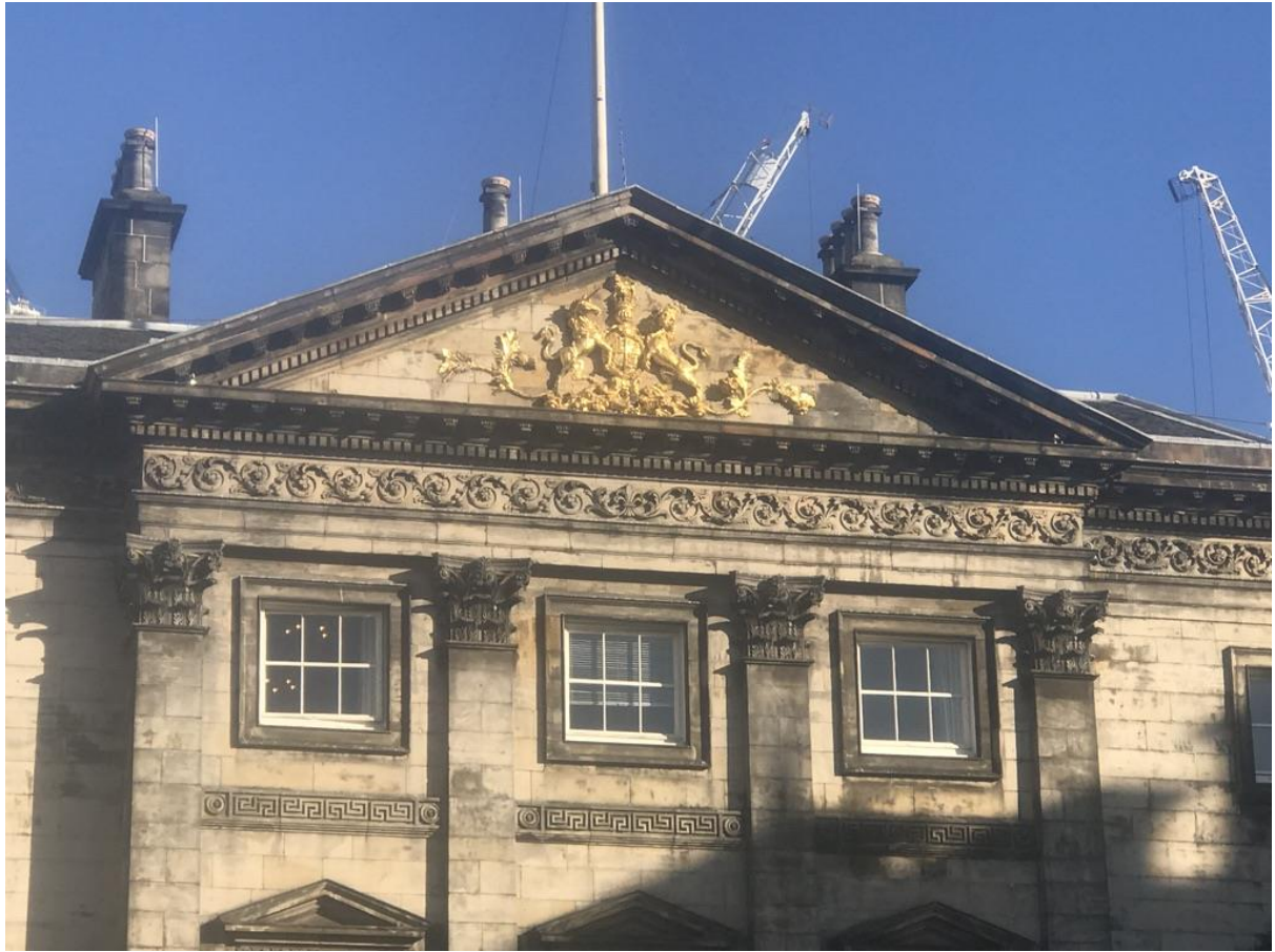
Figure 2.51. Dundas House, Edinburgh. Smooth Ravelstone ashlar, now commonplace in the central belt.
