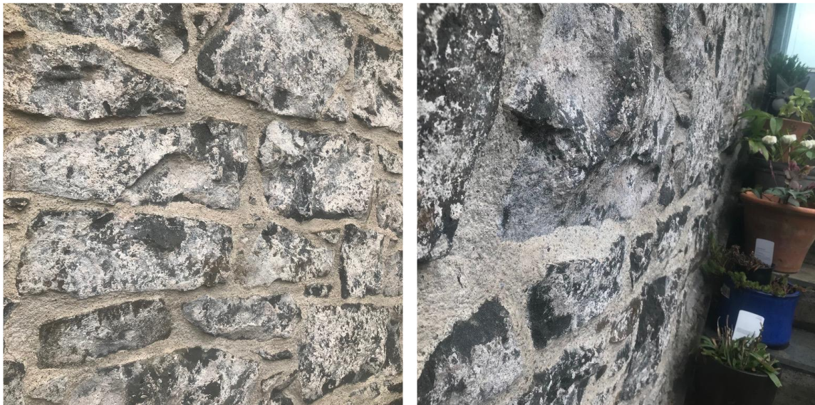
Figure 2.18. Irvine Place, Stirling. The crudely squared basalt, with open ledges.
