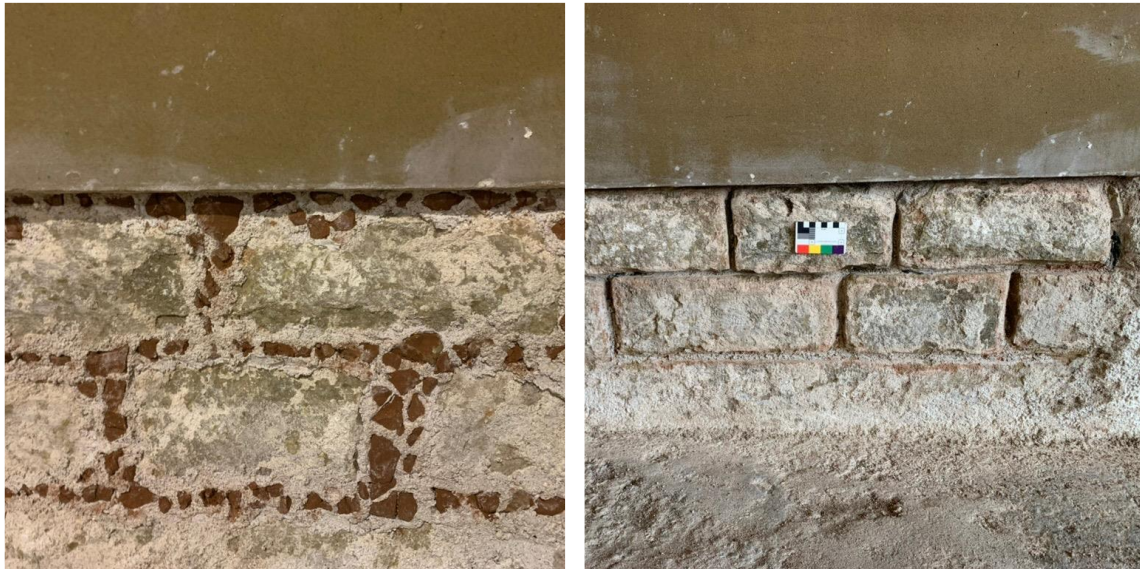
Figure 5.16. Galletting, the latest iteration of the HMM trial that has negated shrinkage at this stage of the process.
