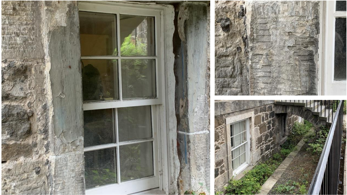
Figure 2.15. Dalgleish Court. Discreet below ground level area, retaining harl and limewash.
