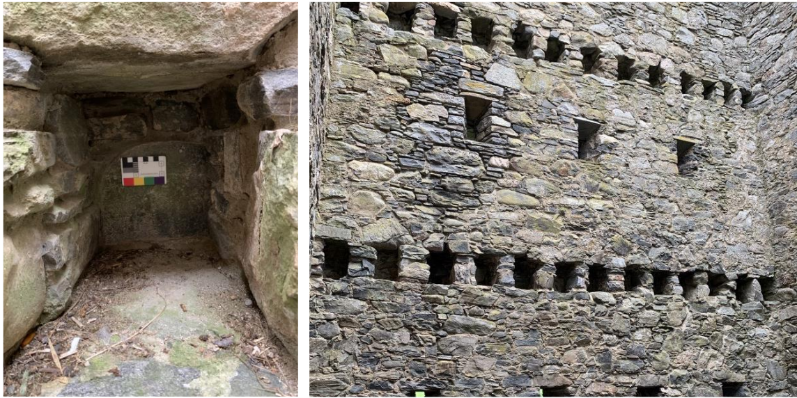
Figure 4.25. Ruthven Barracks: joist slots extending ~400mm into a wall depth of ~600mm.
