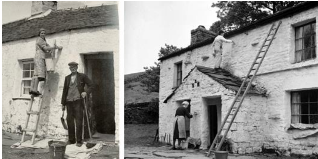
Figure 2.29. Photographic record of limewashing. Left: Alasdair Alpin MacGregor, courtesy of National Museum of Scotland. Right: courtesy of North Yorkshire County Record Office Online Shop, Emily Ward.
