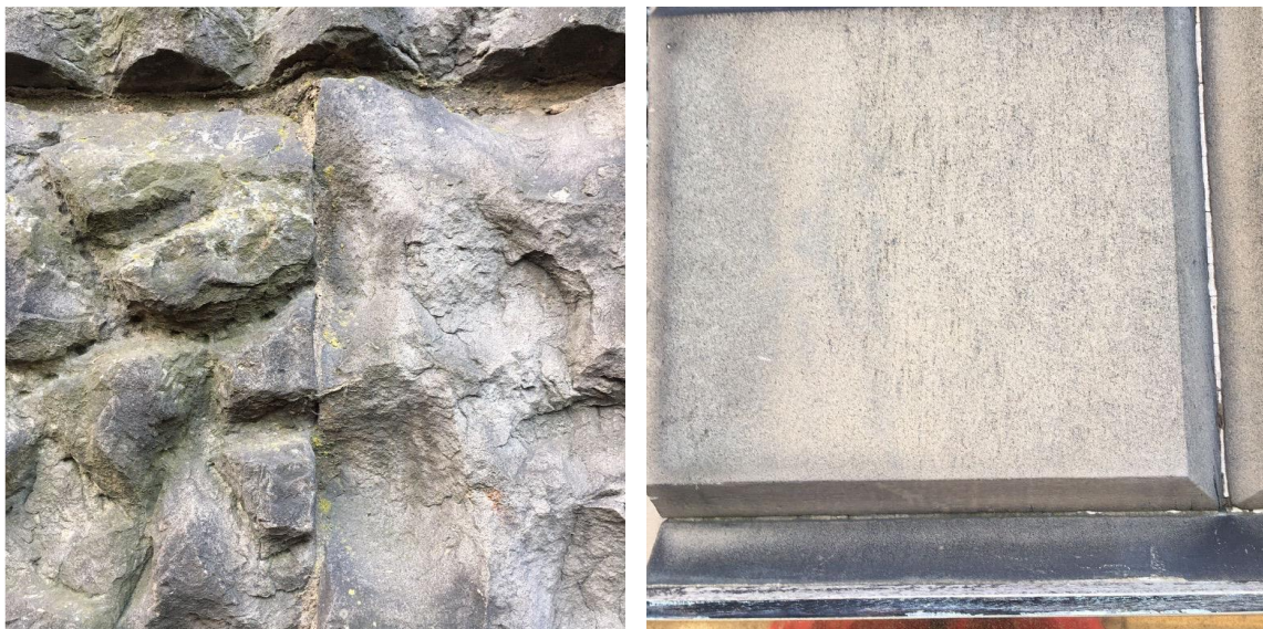
Figure 1.7. Edinburgh bare ashlar with rustic finishes retaining fine joints.
