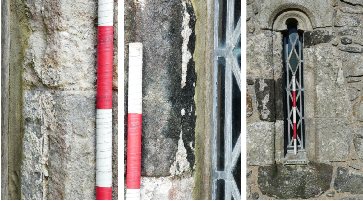
Figure 2.24. St Clement's Rodel. Fine plaster and limewash folding around the decorative components into the glazed area.
