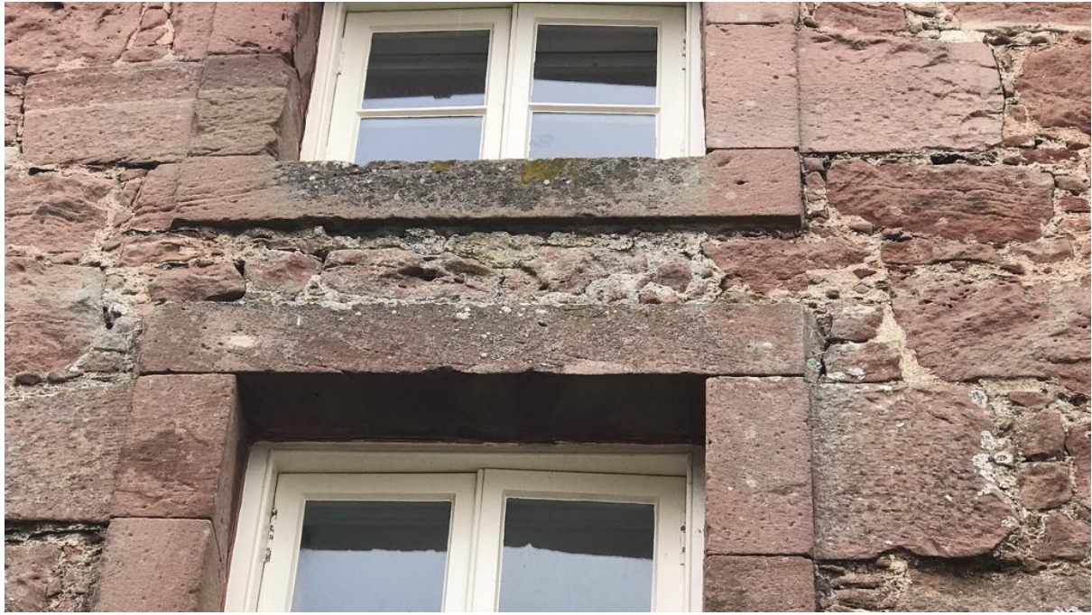
Figure 2.49. Retrospective under sill packing.
