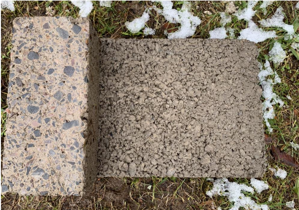
Figure 3.49. A 7.3 N concrete block: left the surface with exposed aggregate and dense binder paste. Right, the as cast open texture with the aggregates with a thin coating of binder paste and interstices between the aggregates.
