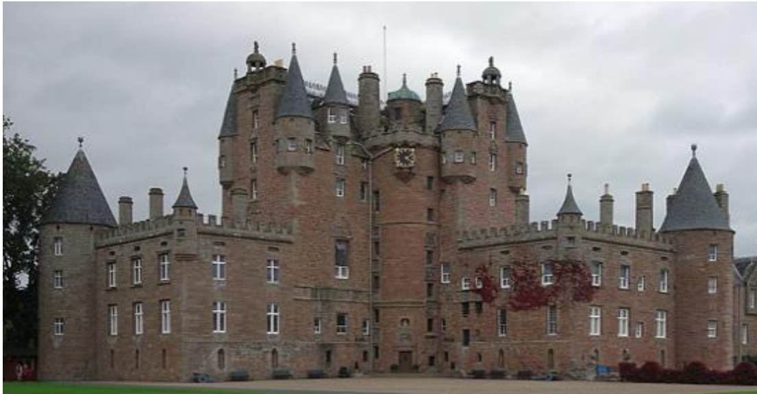
Figure 1.13. Glamis, today. The central towers remain, stripped of harl and the additions built with sawn, coursed rubble.
