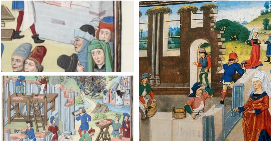
Figure 3.10. Illustrations from Annales historiae illustrium principum Hannoniæ c.1390 – 1396 showing the completion of building surfaces as work proceeds with wall head protection. Image credit Koninklijke Bibliotheek Royale, Belgium. https://uurl.kbr.be/1894866_p345
