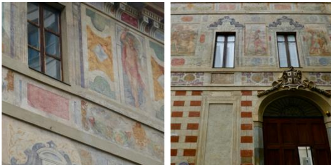
Figure 2.33. 'Marbling, ashlar and colouring', the conserved Palazzoo Scaglia di Verrua, Quadrilatero Romano, Turin, Italy.
