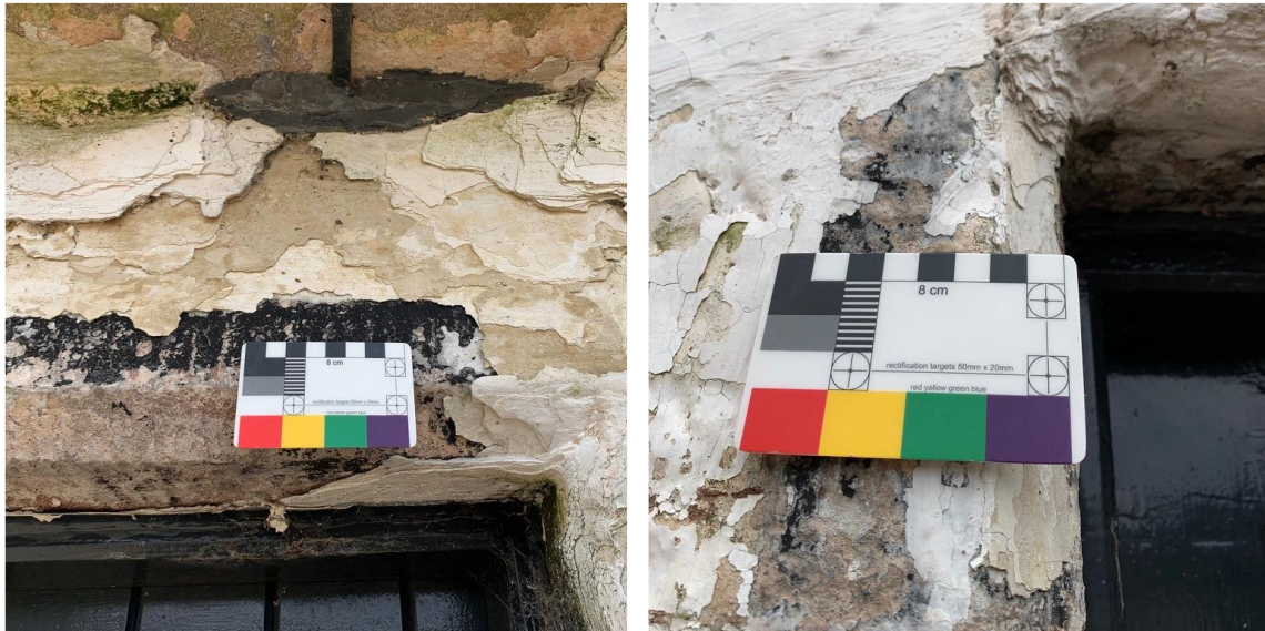
Figure 2.10. Exfoliating multi-layered limewash in sheltered areas.
