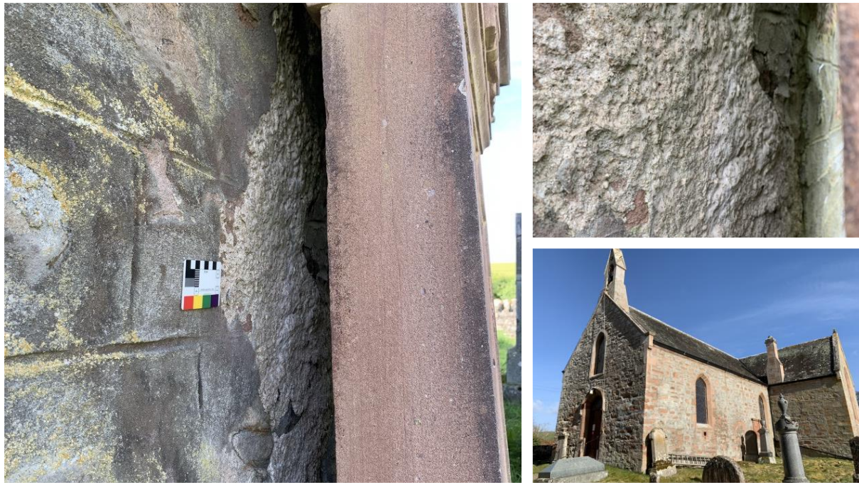
Figure 2.11. Killearnan Parish Church, Ross shire. Outwardly a bare stone Victorian church; evidence from behind grave markers suggested a harled surface.
