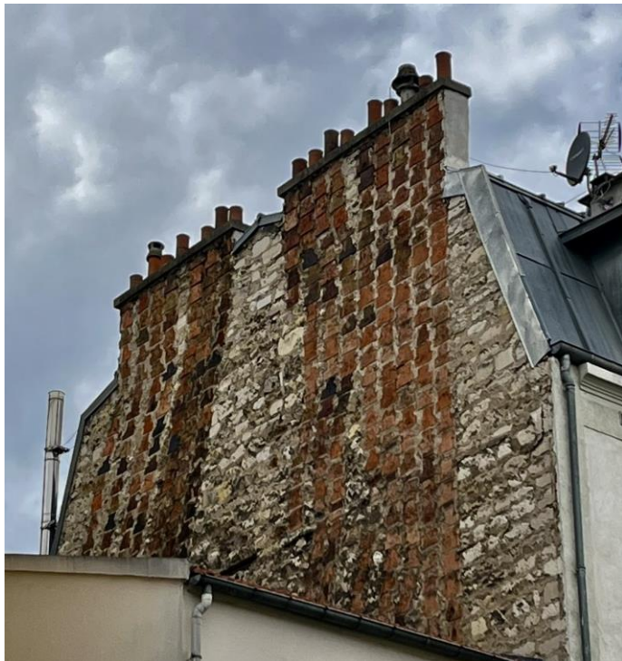
Figure 6.0. Multiple chimney flues in a gable
