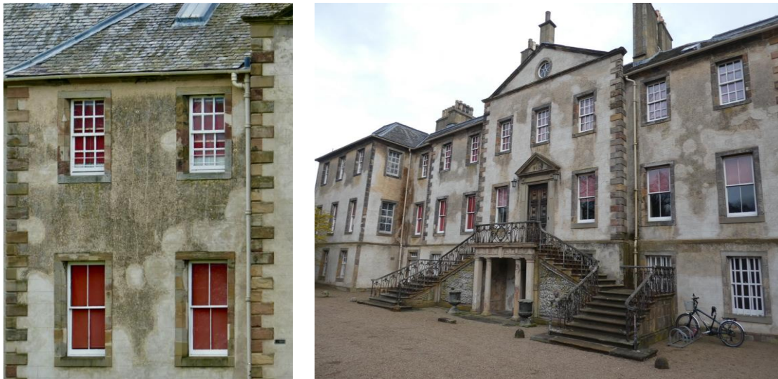
Figure 2.21. Newhails House, Raised margins and raised rusticated quoins.
