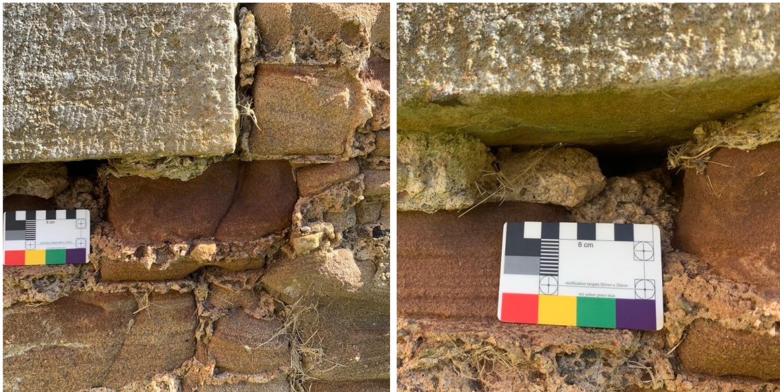
Figure 2.48. Support during the process of levelling sills.
