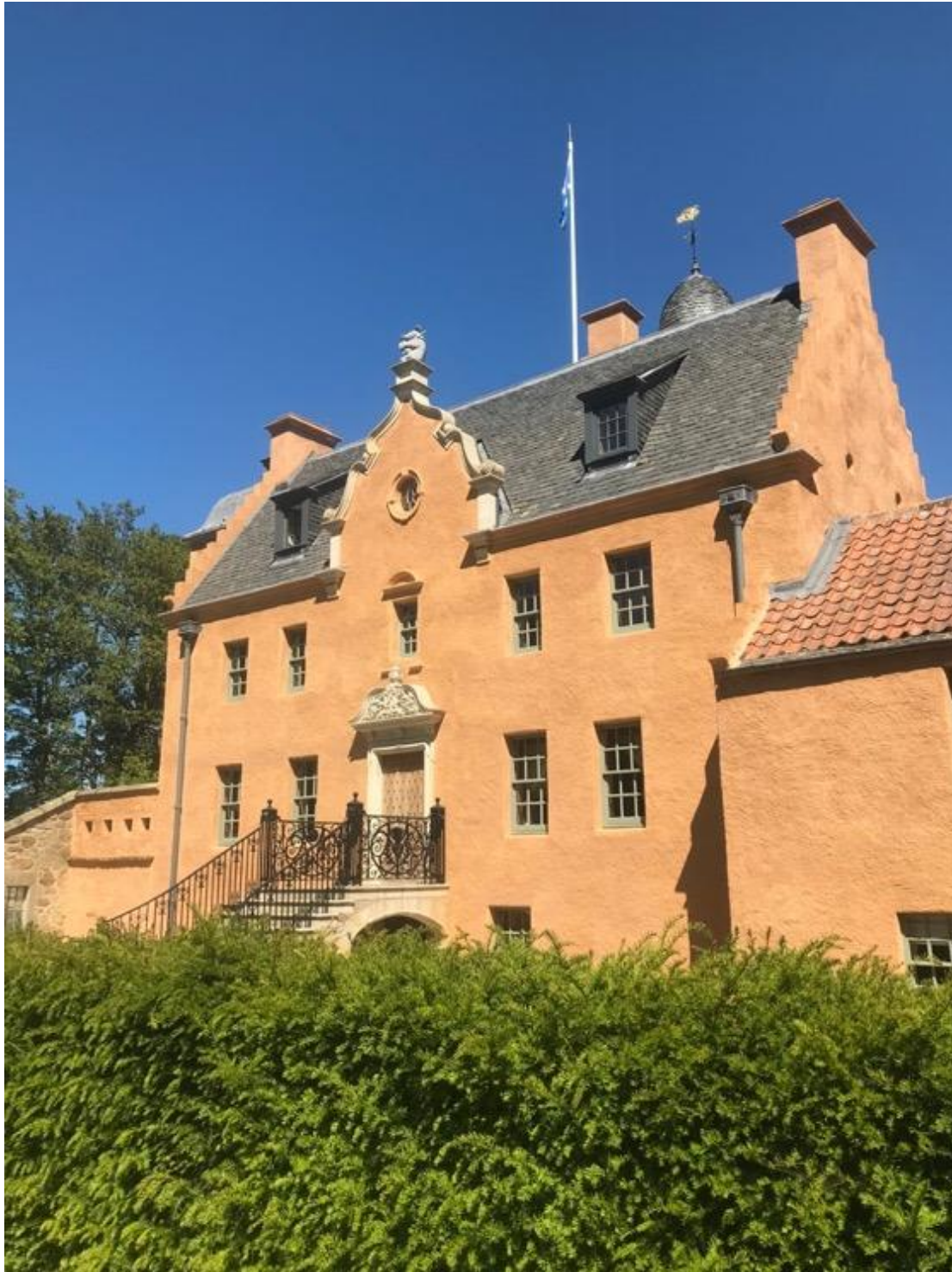
Figure 6.19. Newly harled and limewashed Wormistoun House, Crail, Fife. New work and old blended, protected, seamless and in contemporary world still demonstrating the 'arrival' of the current owners.
