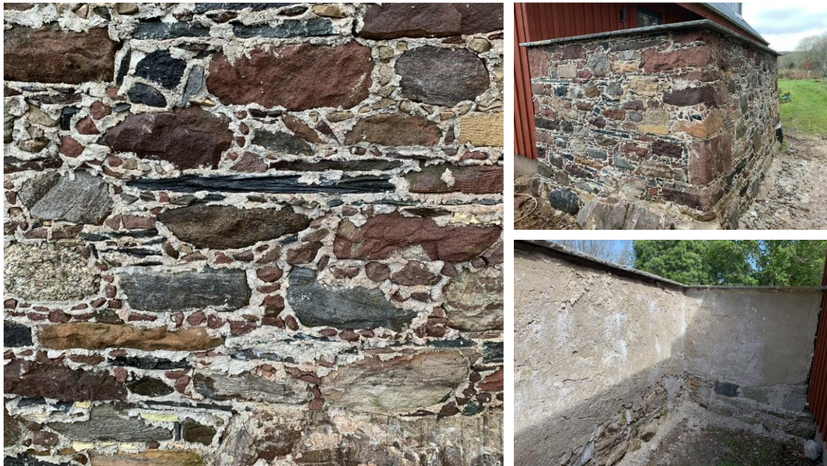
Figure 3.54. The Poyntzfield wall, large and small stones, flagstone capped.
