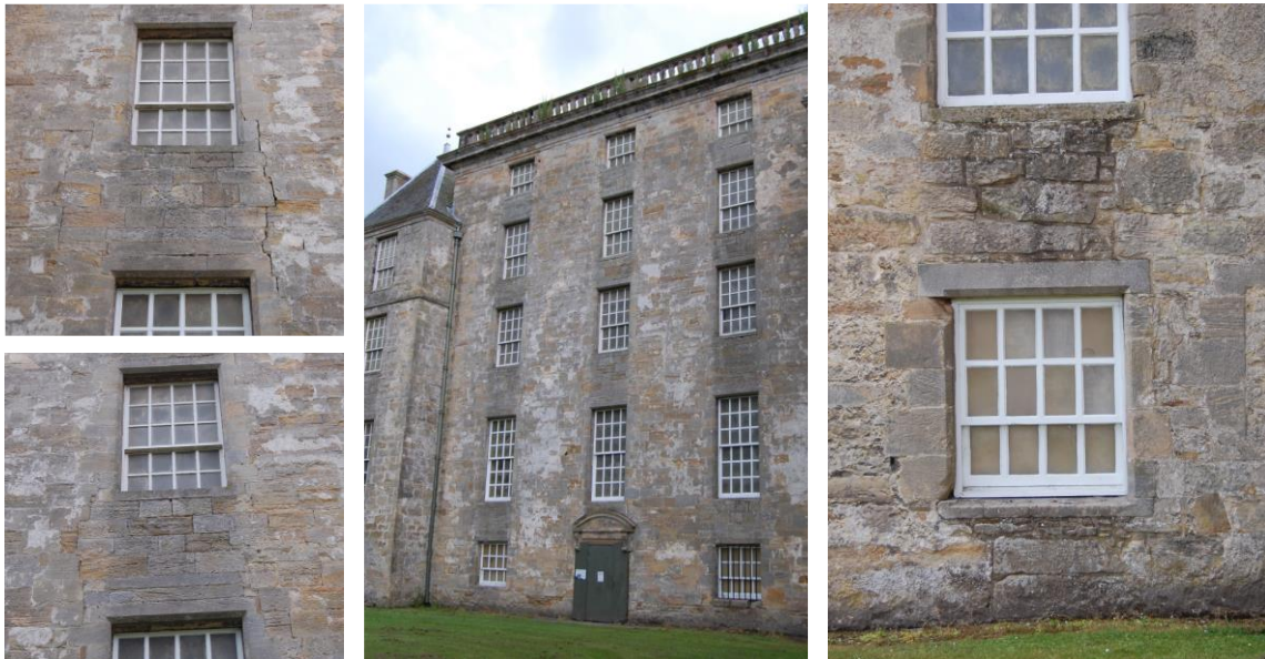
Figure 2.47. Kinniel House, Bo'ness, c.1553. Altered in the seventeenth-century to accommodate newly fashionable sliding sash windows.
