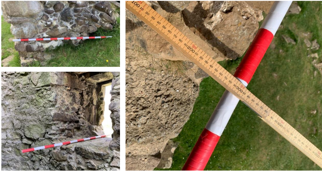
Figure 2.37. Wall widths at Ardvreck Castle.
