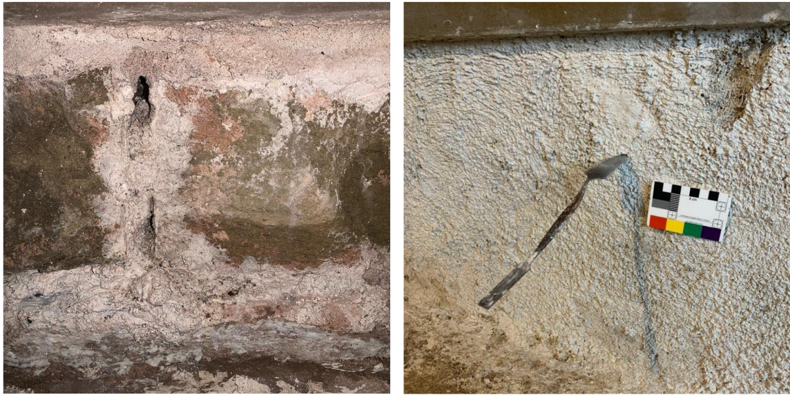
Figure 5.17. Breakdown (left) and softness (right) of the HMM harl and building mortars after repeated PD runs.
