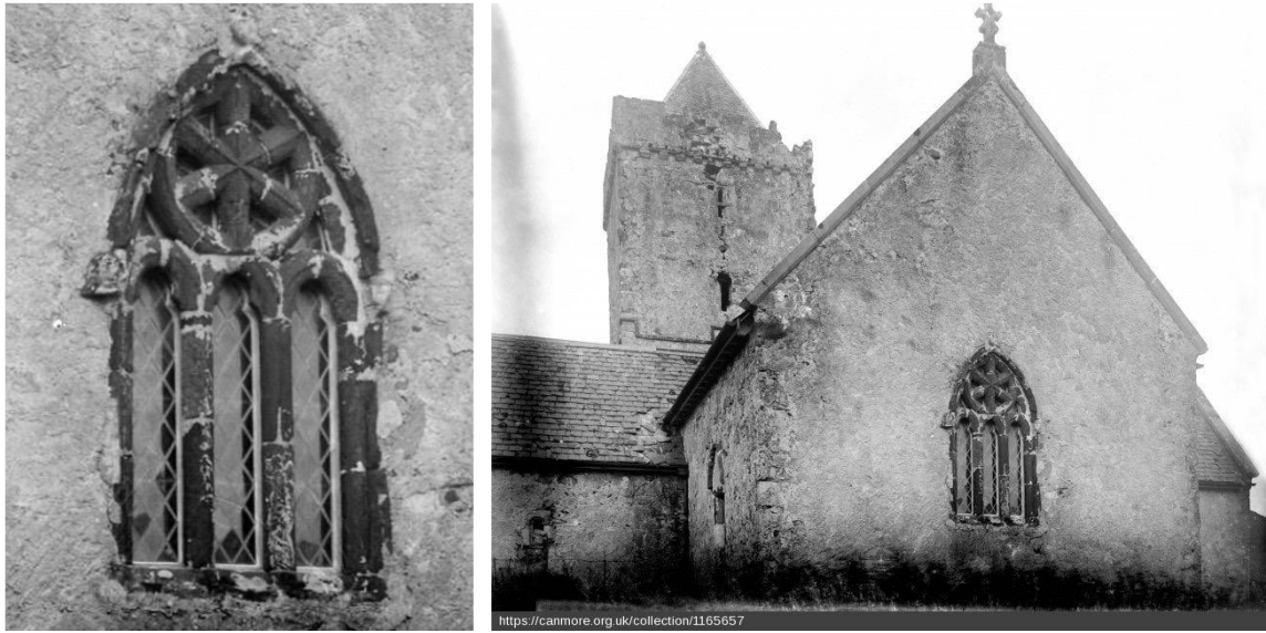
Figure 2.1. St Clement's, lancet window with extant plaster/limewash ( https://canmore.org.uk/file/image/1165657 ).
