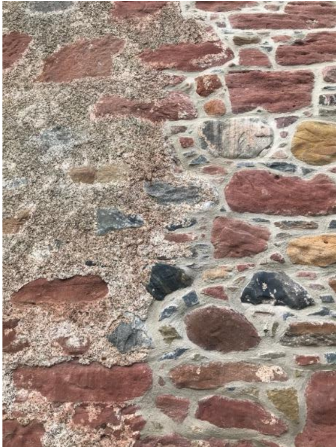
Figure 6.18. New repointing work to worn sneck harl using a style universal throughout Scotland.
