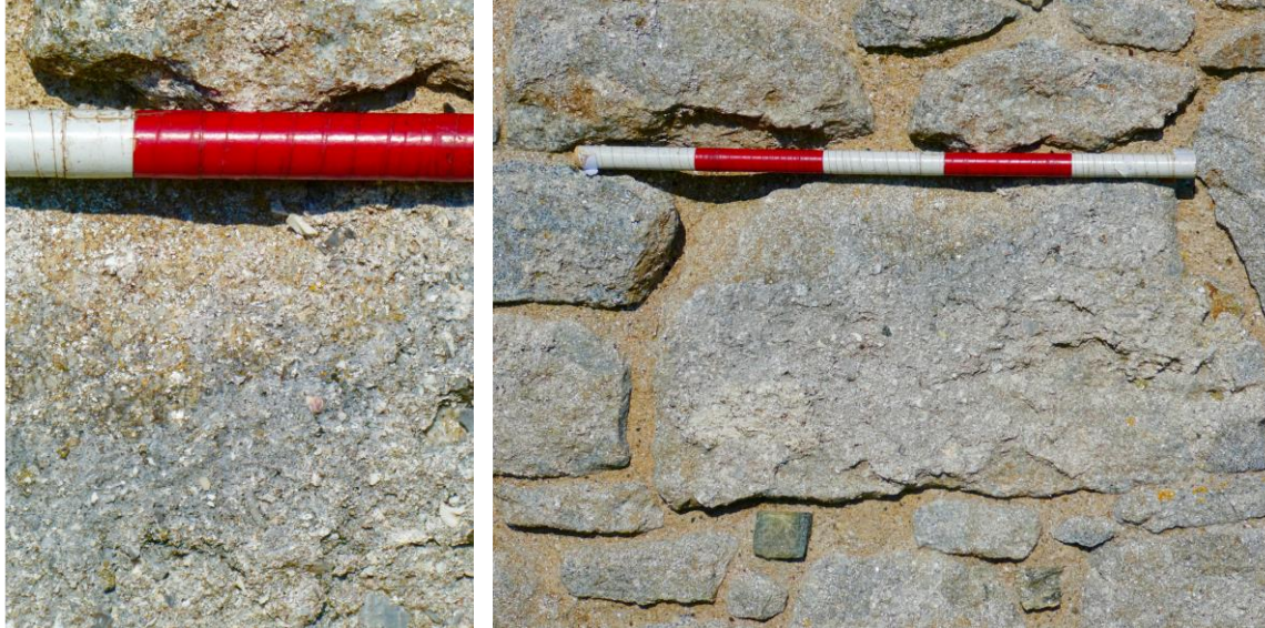
Figure 2.8. Left: Detail of 16 th century marine harl at Rodel, Harris. Right: The same harl in context with the stone, demonstrating the importance of close scrutiny to identify the difference between stone and harl when the wall is completely covered in biological growth.
