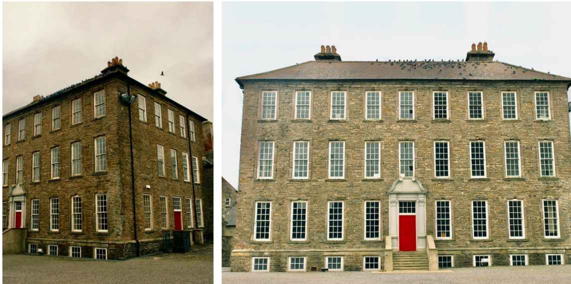
Figure 4.0. Darmer House, Roscrea Co. Tipperary, Ireland, showing the multiple stacking of windows on adjacent elevations (Image credit Tom Marnell).
