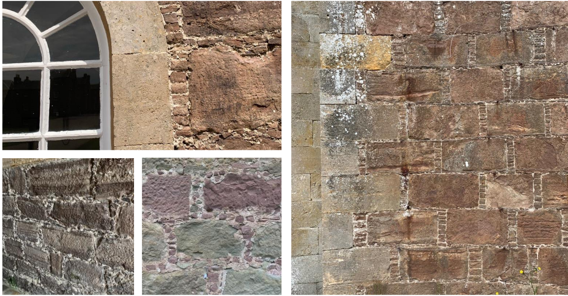
Figure 5.15. Eighteenth-century cherry-cocking/galletting used between the blocks to reduce water penetration.
