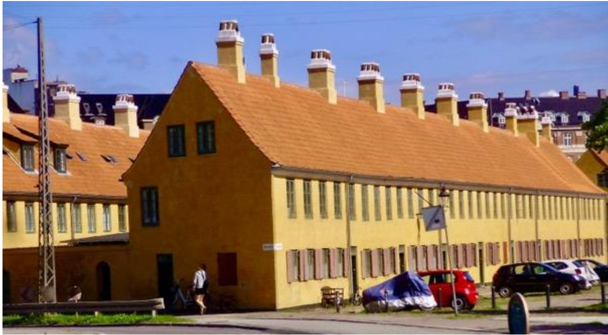
Figure 6.8 Copenhagen, Denmark. Former naval quarters, Plastered and limewashed. Image credit Dr Nina Baker.
