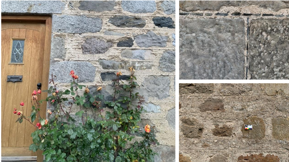
Figure 2.63. Formal, ruled out pointing styles.
