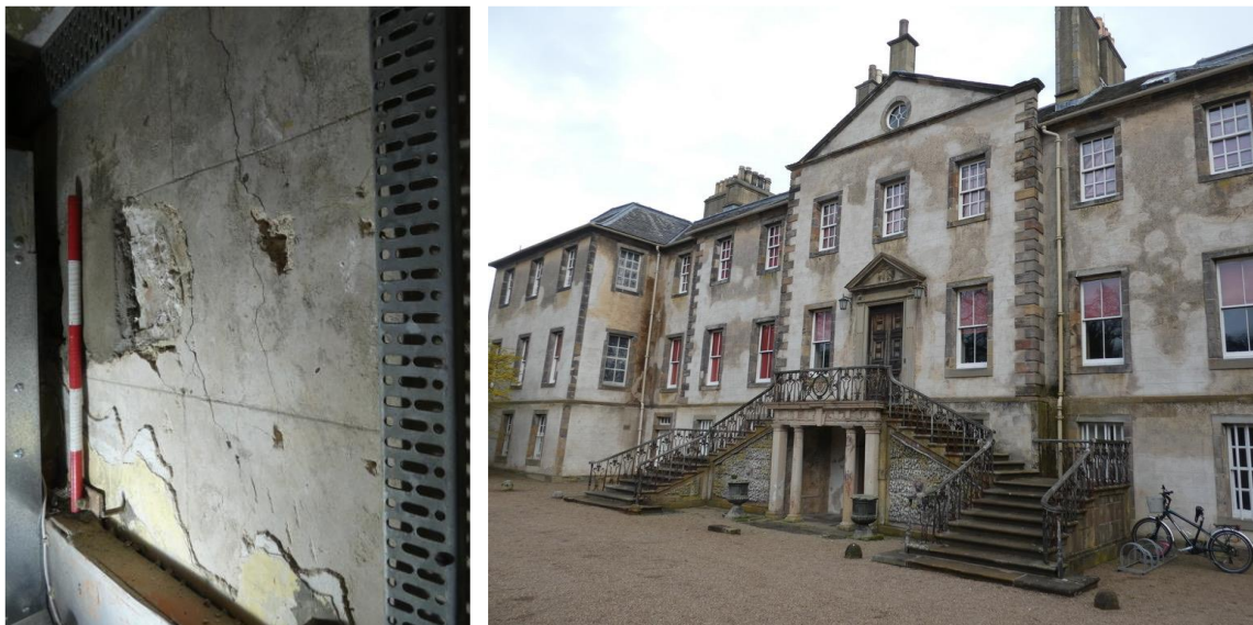
Figure 2.13. Newhailes House, Musselburgh, East Lothian. Fully plastered and lined out 'ashlar' Left the basement area where the work of James Smith c.1686 was enclosed within the later work of William Adam c.1721.
