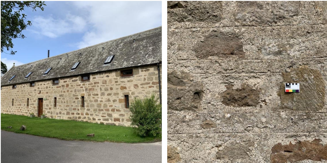
Figure 2.66. The Granary, sneck harled and ruled out.
