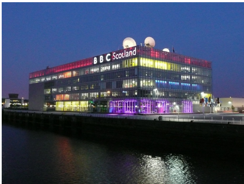
BBC Scotland HQ on the banks of the Clyde in Glasgow. John Dee, CC BY-SA
