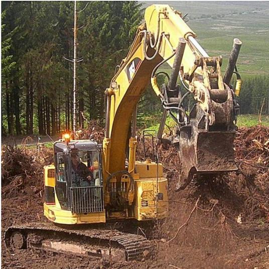
Figure 5-1: Stump extraction.
