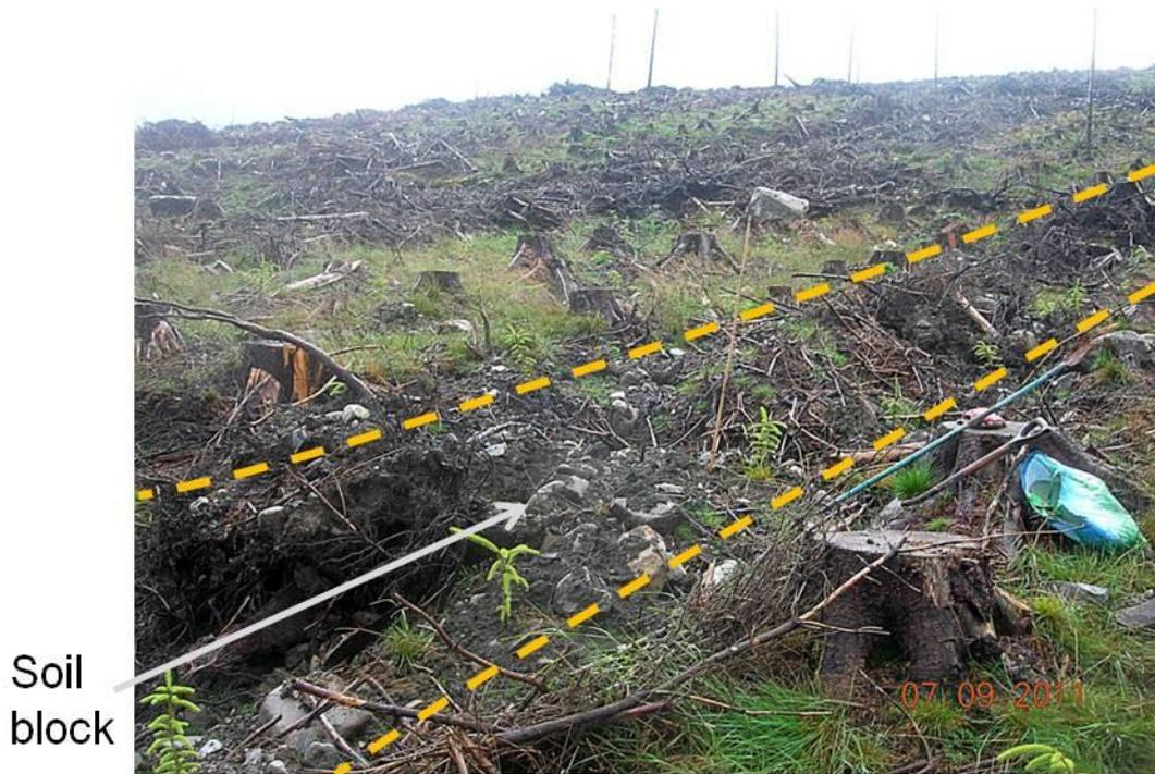
**Figure 2-17: Spoil trench refilled with displaced stumps, brush and unused spoil.**
