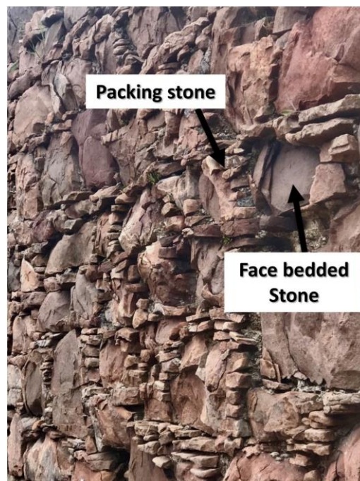
Figure 6.4 - Face bedded Torridonian Sandstone at Tanera Mòr Herring Station. Packing stones sit proud of the larger face bedded block. Image courtesy of Timothy Meek
