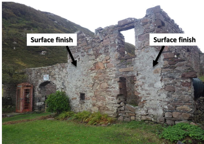
Figure 6.6 - Tanera Mòr Herring Station building, comparative lack of Torridonian Sandstone weathering seen on areas of the building that have a surface finish. Image courtesy of Timothy Meek
