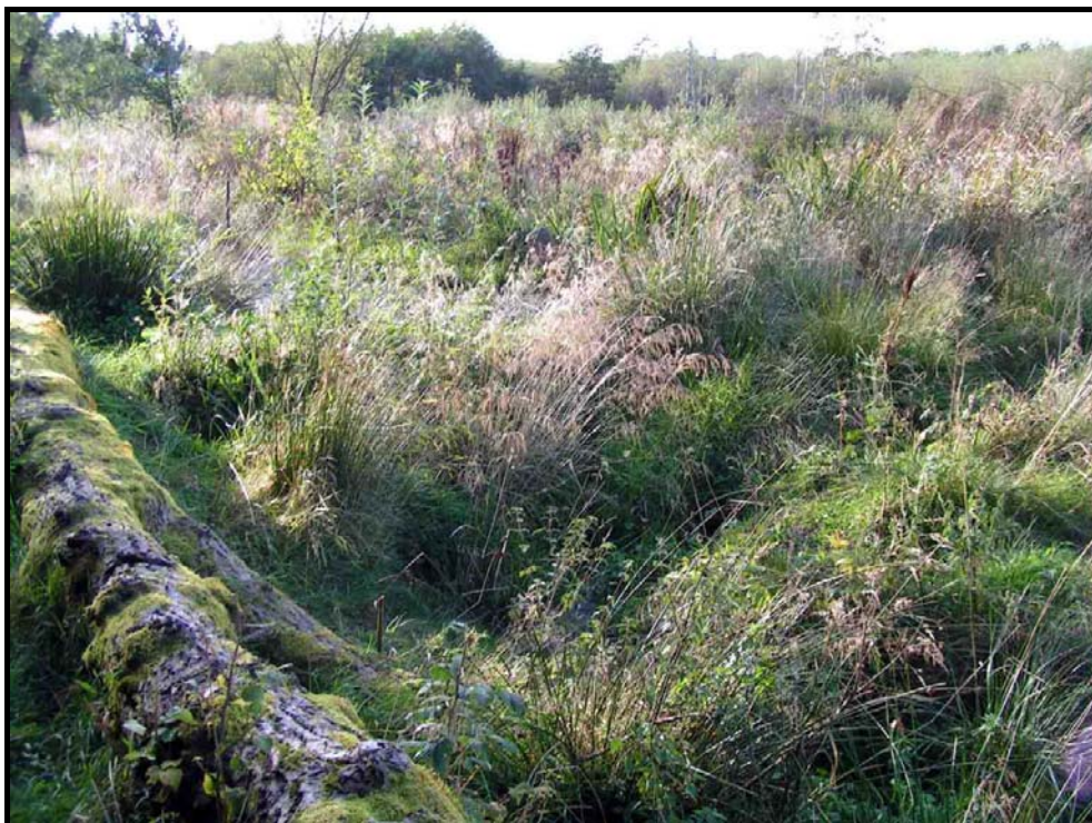
Figure 6.10b Dam 1 at the Stream Site in September 2004, showing vegetation cover including abundant willow regrowth from branches incorporated into the structure.
